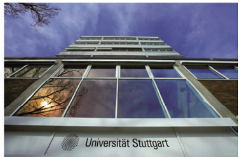
Modern buildings on the Campus Vaihingen
