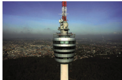
Television Tower – Landmark of the city and the first in the world built of ferroconcrete
